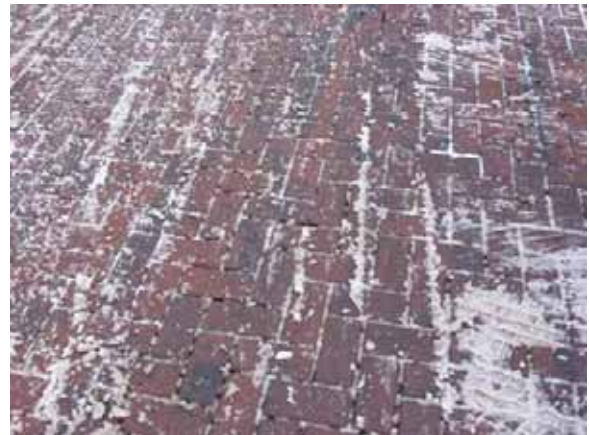
Figure 16: Snow cover after plowing but before sun begins to warm up pavement.
